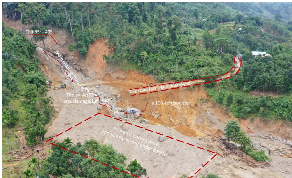
Figure 3. TraLeng debris fan and damaged infrastructure (UAV picture).
